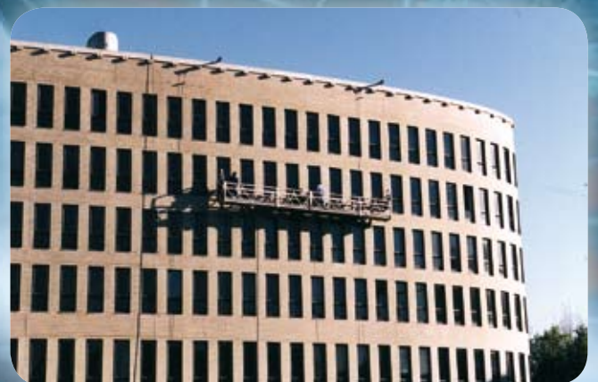
ALTA platform 8 m with 2 suspensions PORTAFIX, Brussels
