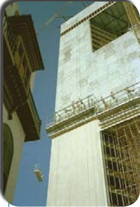
Double decked ALTA platform delivered with an overhead crane for load handling (marble plates) and personal lift, Saudi Arabia
