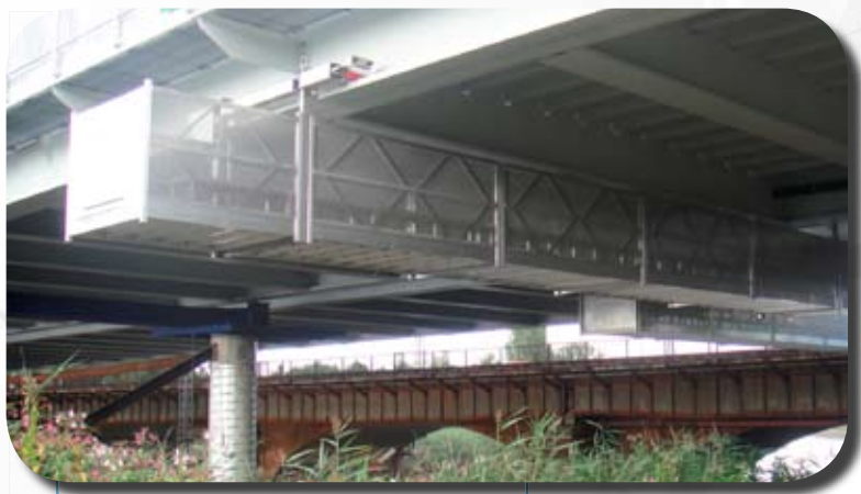
15 m gantry for bridge repair work, Belgium
