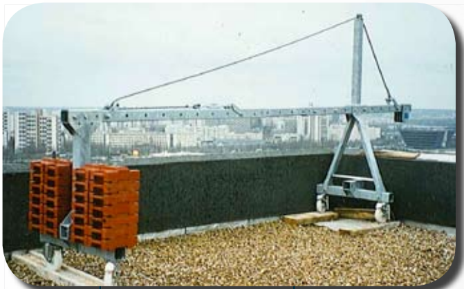
Low-rise building, France
