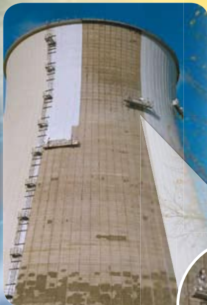
3 ALTA platforms 6 m, cooling tower, Belgium
