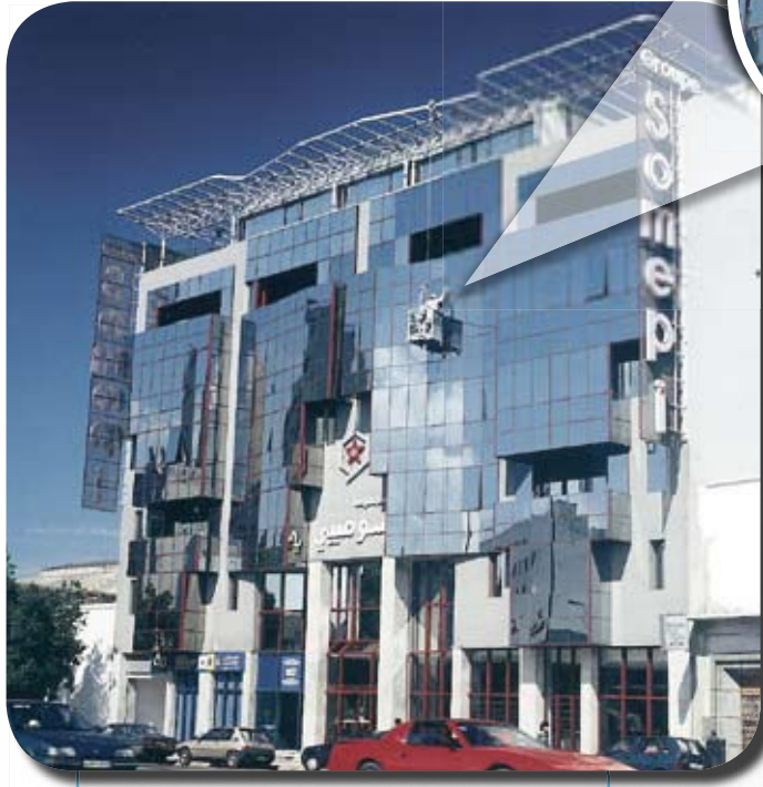
Permanently attached SOLO platform to monorail for cleaning, Casablanca
