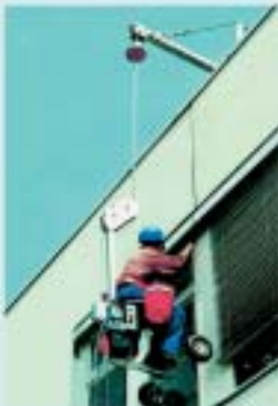
Access cradle for repair work
