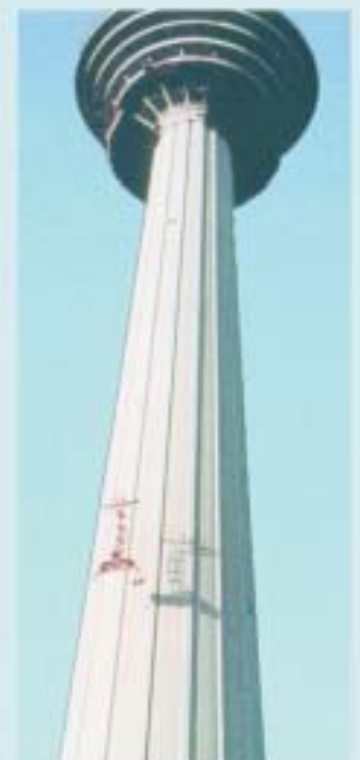
TIRAK® installed above the load under the upper part of the tower
