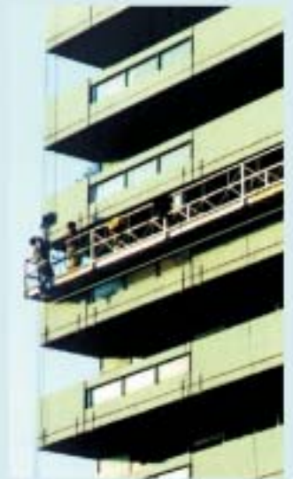
Access cradle for facade refurbishment
