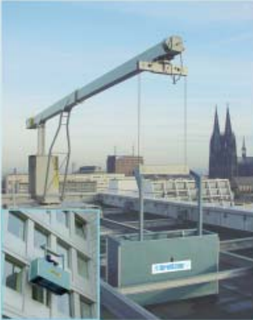
Facade inspection installation with moving trolley on roof – the TIRAK® is installed on the centralised control platform.
